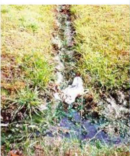
Failing Septic Systems
